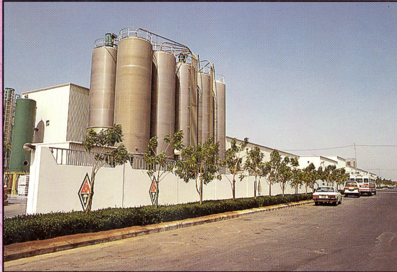
Ten silos for material distribution before mixing.
